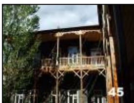
45. Left: Aslamazian Sisters Gallery , 1880-1890. Rebuilt. This pure “Belle Époque” building of black tufa shows itself with clean lines, neat joints and smooth facade. Note the sun symbol on the façade. There is a courtyard in the back with a garden and rebuilt porch. The building houses the Aslamazian Sisters Museum (see Art).
