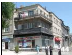
44. At Left corner, constructivist style building erected in 1930. The balconies are original and show an early attempt to combine modern and older style.
