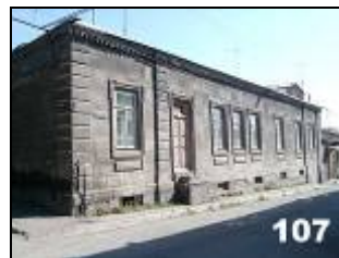
107. Left Opposite corner: Stone Dwelling House , 1880-1890.
