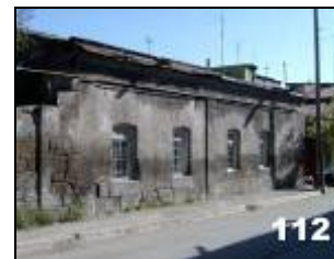
112. Left three doors down: Dwelling , 1860-1880.
