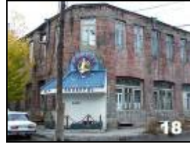
18. Cattycorner Right: Jrahars Fish restaurant inside 1890 building. Note the beautiful window design in the wall.
