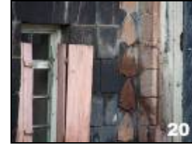
20. Left next building: dwelling, shop , 1860-1880. Black and red tufa in classic style. You can see where the main gate has been walled over, the metal one cut through the older wall. The windows have some of the original wooden shutters. This style of closing off windows is a classic feature of Old Giumri architecture. Note the far right corner of the building: the red tufa is shaped like shovels, possibly indicating the type of work own there (blacksmithing, farm implements).
