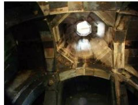
When it was decided to add a two-story **bell-tower**, both structures were rebuilt, the construction done in two stages; eight wall abutments were added to support a new stone roof held by two pairs of cross-arches that covered the new library cruciform superstructure. The second floor was halted (due to Mongol incursions in the area begun in 1238), with barely two rows of stone and half columns completed before construction stopped.
