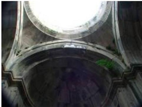
The arch distributes the force of the wall away from the window hole, allowing it to remain open. Domes certainly depended on their support walls and abutments, but they also served to spread weight evenly across the substructure, as well as tying the walls together, preventing them from leaning outwards. Without the dome, S. Grigor's walls were susceptible to both the elements and to their natural outward force, in effect pulling the walls away from each other.
