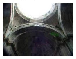
The arch distributes the force of the wall away from the window hole, allowing it to remain open. Domes certainly depended on their support walls and abutments, but they also served to spread weight evenly across the substructure, as well as tying the walls together, preventing them from leaning outwards. Without the dome, S. Grigor's walls were susceptible to both the elements and to their natural outward force, in effect pulling the walls away from each other.
