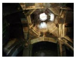
When it was decided to add a two-story *bell-tower*, both structures were rebuilt, the construction done in two stages; eight wall abutments were added to support a new stone roof held by two pairs of cross-arches that covered the new library cruciform superstructure. The second floor was halted (due to Mongol incursions in the area begun in 1238), with barely two rows of stone and half columns completed before construction stopped.
